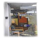
Glass originally was not designed to resist windblown debris, explosions, vandalism, forced entry or anything else that can put stress on it. When broken, this glass would produce lethal shards or fall in large pieces. To prevent this, legislation was passed in the 70's mandating the use of tempered glass. The mandates however only cover particular areas such as: floor to ceiling windows; glass doors; panes of glass next to doors; and glass areas next to heavy pedestrian traffic.
