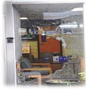
Glass originally was not designed to resist windblown debris, explosions, vandalism, forced entry or anything else that can put stress on it. When broken, this glass would produce lethal shards or fall in large pieces. To prevent this, legislation was passed in the 70's mandating the use of tempered glass. The mandates however only cover particular areas such as: floor to ceiling windows; glass doors; panes of glass next to doors; and glass areas next to heavy pedestrian traffic.
